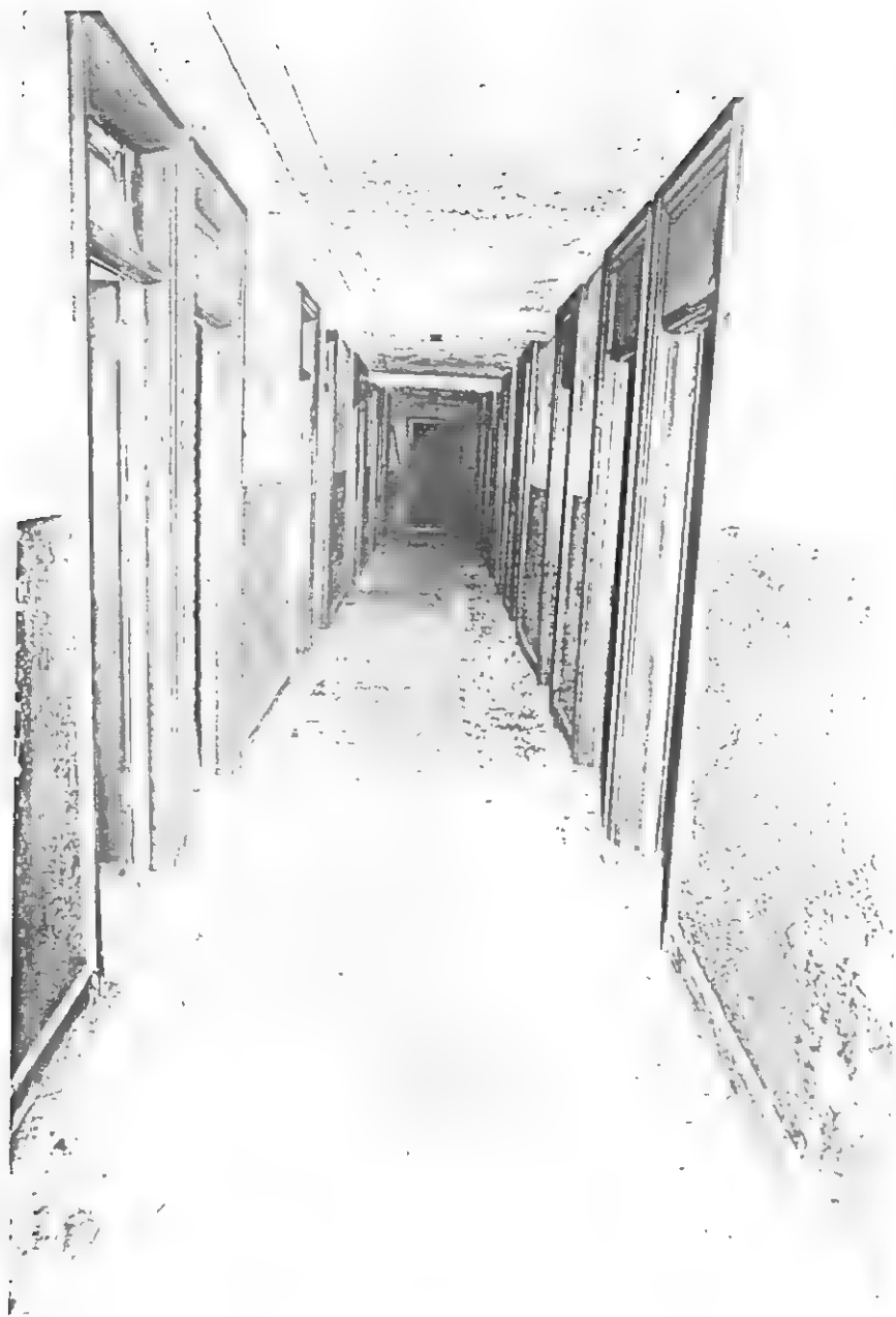
Typical view of YMCA Building hallways on the third and fourth floors.
